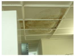
Figure 1 Ceiling tiles damaged by water adjacent to seed drying room
